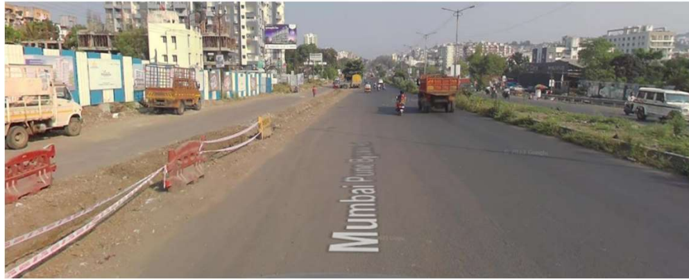
Survey location 1 -Mumbai Pune Bypass Road (60 M Wide )
