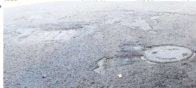
Photos of Existing drainage & storm water chamber
